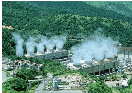
Geothermal Power Plants
