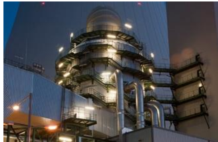
Environmental Plants SCR (DeNOx) Systems / Flue Gas Desulfurization
